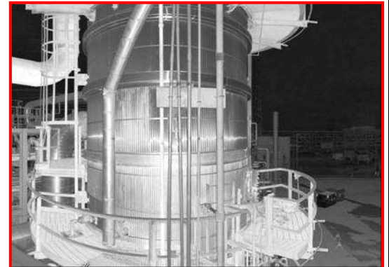
Quantapoint Laser Image (Not a Picture) Each Point is a Measurement
