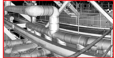
Quantapoint Laser Image (Not a Picture) Each Point is a Measurement
