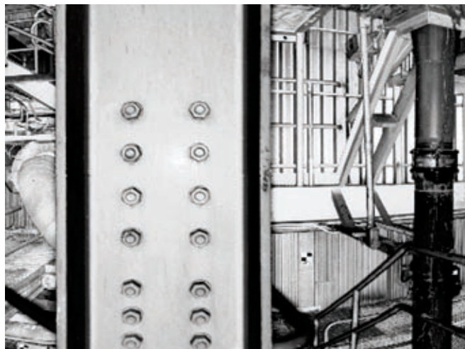
FIG. 3 Zooming into the laser documentation shows fine details that are captured, including threading on bolts.
