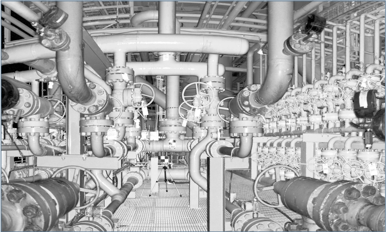
Actual laser scan (not a photo) of an offshore facility, from which dimensions, pipe sizes, tie points and other information can be extracted.
