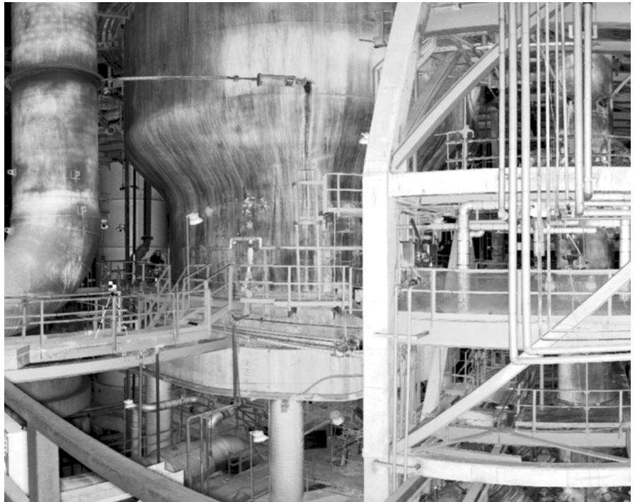
1. Shell game. Shell Oil hired Quantapoint to create laser images of five of its refineries to facilitate upgrading the emissions performance of Shell's generating units. Shown is a laser image of the equipment and pipes at one of the facilities in Houston. Courtesy: Quantapoint Inc.
