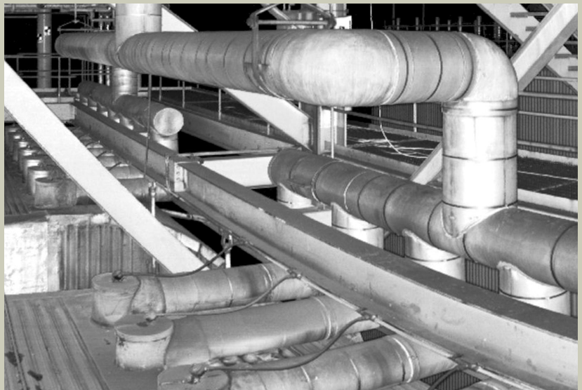
3. Prettier than a picture. In this laser scan (not a photograph) of power plant piping atop a baghouse, each point in the image represents a highly accurate measurement. Courtesy: Quantapoint Inc.
