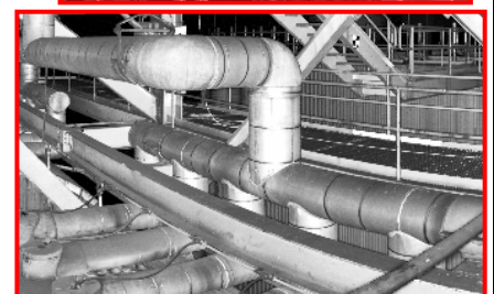
Quantapoint 2D Laser Scan ( not a Picture) Each Point is a Measurement
